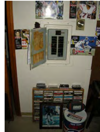
Accessible unit circuit breaker panel (typical) compliant with UFAS height and reach guidelines.
