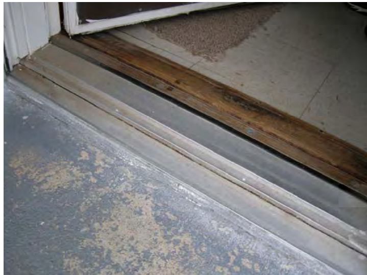
Secondary accessible unit egress is non-compliant with UFAS obstruction guidelines.
