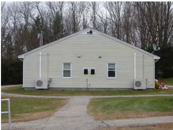
Typical building end view. Showing typical split-system heat pumps exterior components and kitchen exhaust vents
