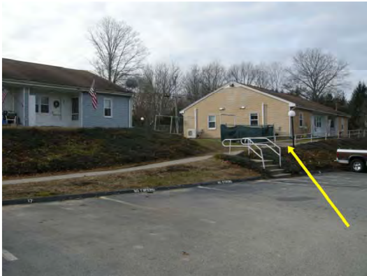
Wheelchair ramp at second terrace level. Slope is in compliance but lack of landings and handrail are not.
