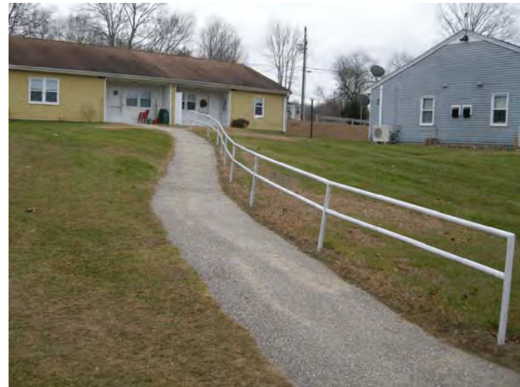
Wheelchair ramp to upper terrace area. Slope and hand rail are not compliant with UFAS guidelines.
