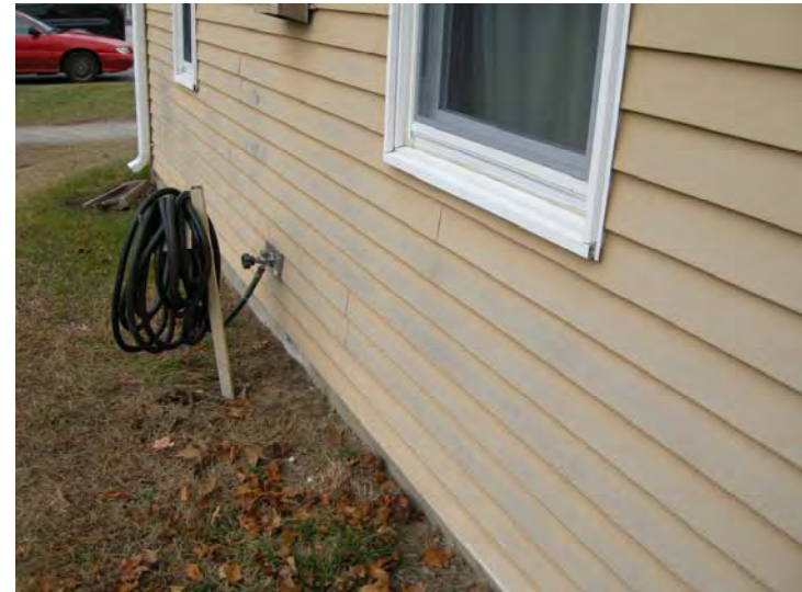
Close up of the aluminum siding showing age related wear
