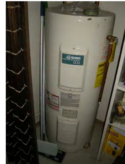
Typical dwelling unit electric domestic hot water heater.
