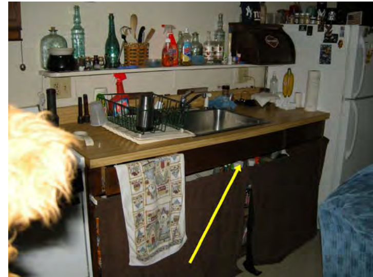
Typical accessible unit kitchen. Note shelving under the sink blocking knee clearance space.
