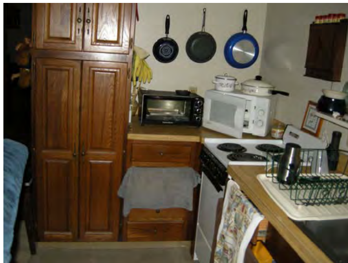
View of accessible unit kitchen storage cabinet. Note lack of work area with under counter knee space
